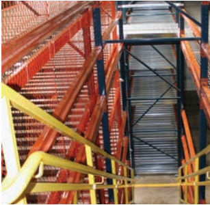
Netting should be installed along stairways
