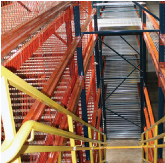
Netting should be installed along stairways
