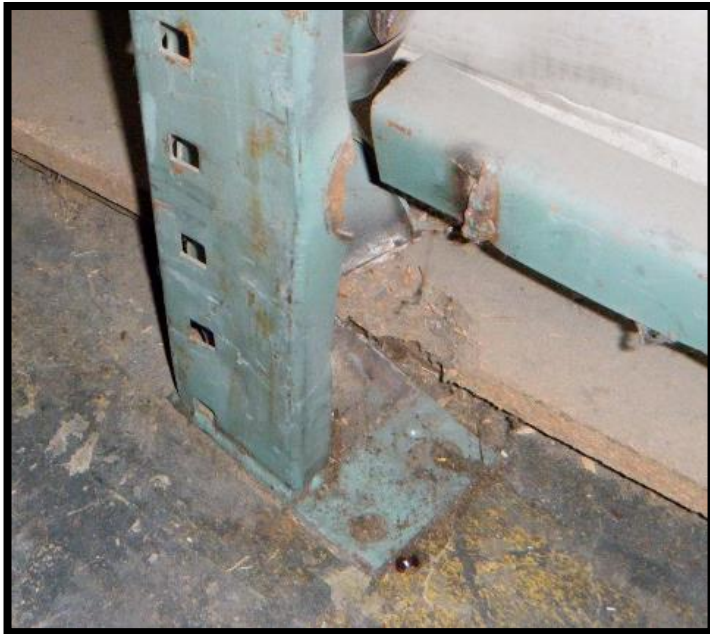
Sheered footplate with missing anchors
