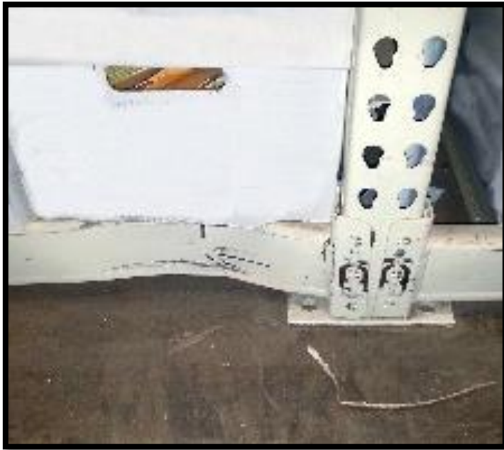
Beam damage with missing safety clips
