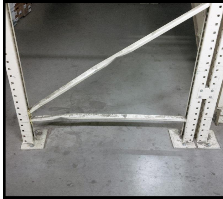
Horizontal & diagonal strut deflection
