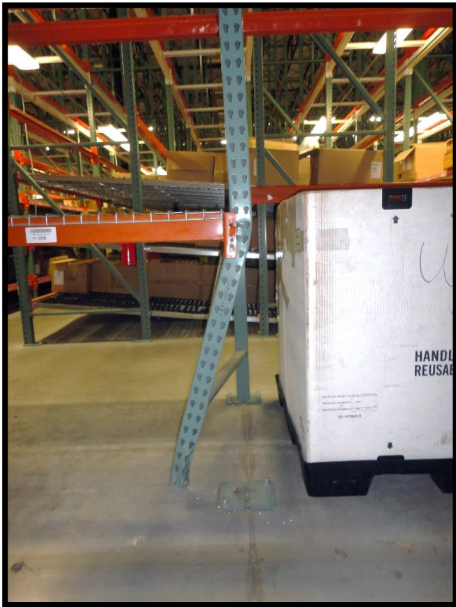
Damaged column
