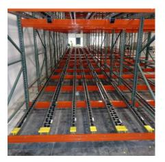
Rack supports inclined rollers or wheels that allow pallets to glide from the back (loading) aisle to the front (picking) aisle. Brakes can be included for speed control. These gravity systems provide excellent volume utilization.
