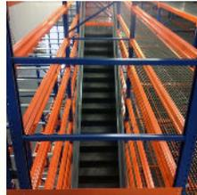
**Flooring:** several options available resin board, corrugated decking, bar grating, open steel planking, and concrete. Each type of floor is better suited for different functions and operational features.
