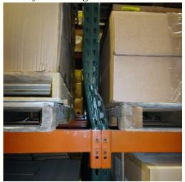
Horizontal and Diagonal Strut Damage: Broken welds, missing braces, or braces with rips, tears or deflection beyond acceptable limits.
