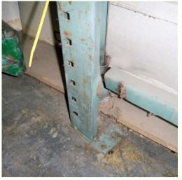
Leaning Frames: A minimum plumbness and straightness (both cross and down aisle) of 1/2"per 10' of height. Missing or Damaged Components: Wall ties, cross-aisle ties, crossbars, beam safety pins, wire mesh decks or pallet stops.
