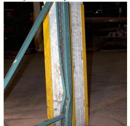
Footplate Damage: Sheared or twisted beyond acceptable limits.
